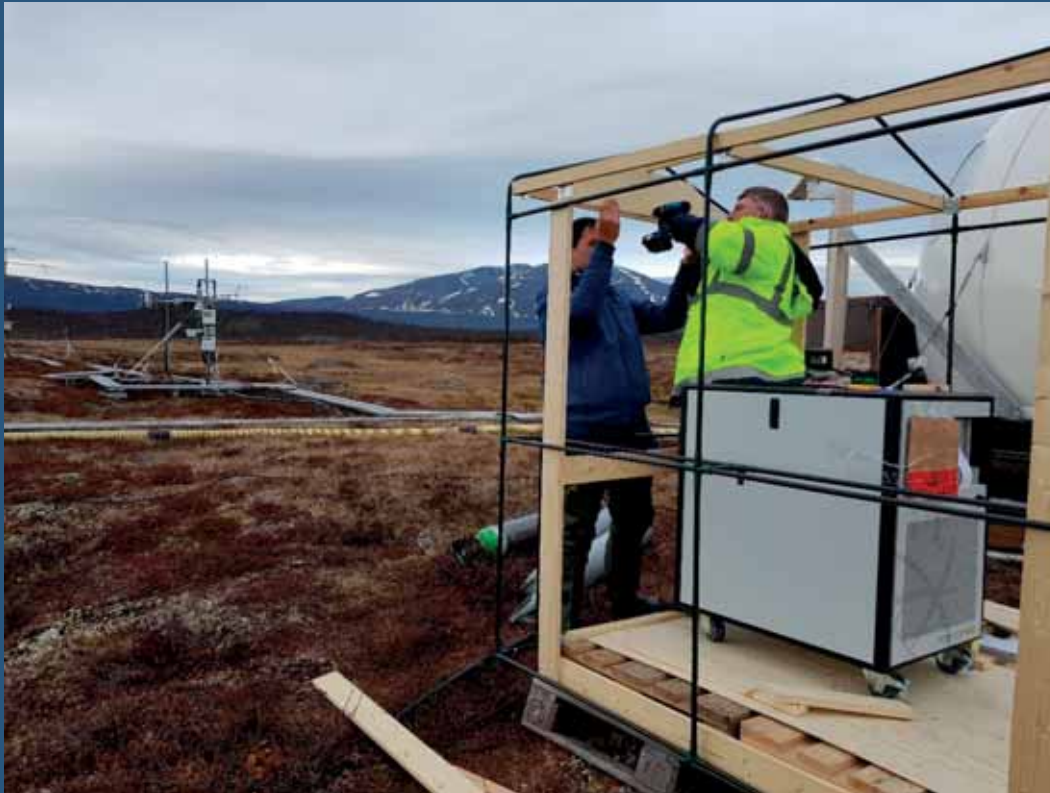
Building a hut around a PTR-TOF-MS instrument coupled to an eddy covariance mast to the left in the photo. Photo: R. Rinnan.
